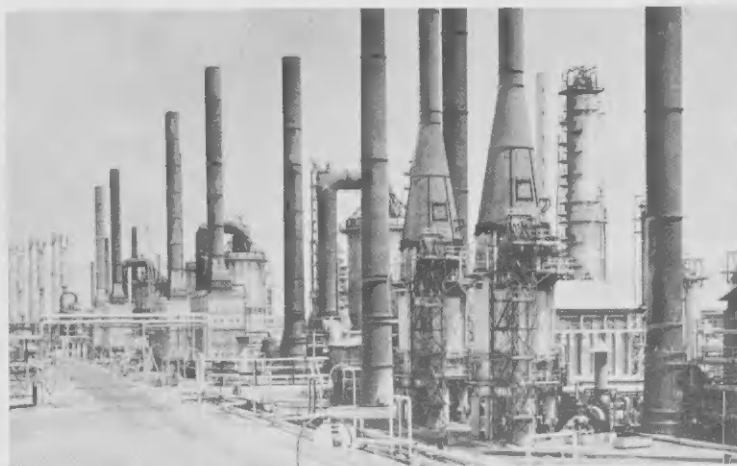
View of Pipestills 5, 6, 7, 8, 9 and 10.
